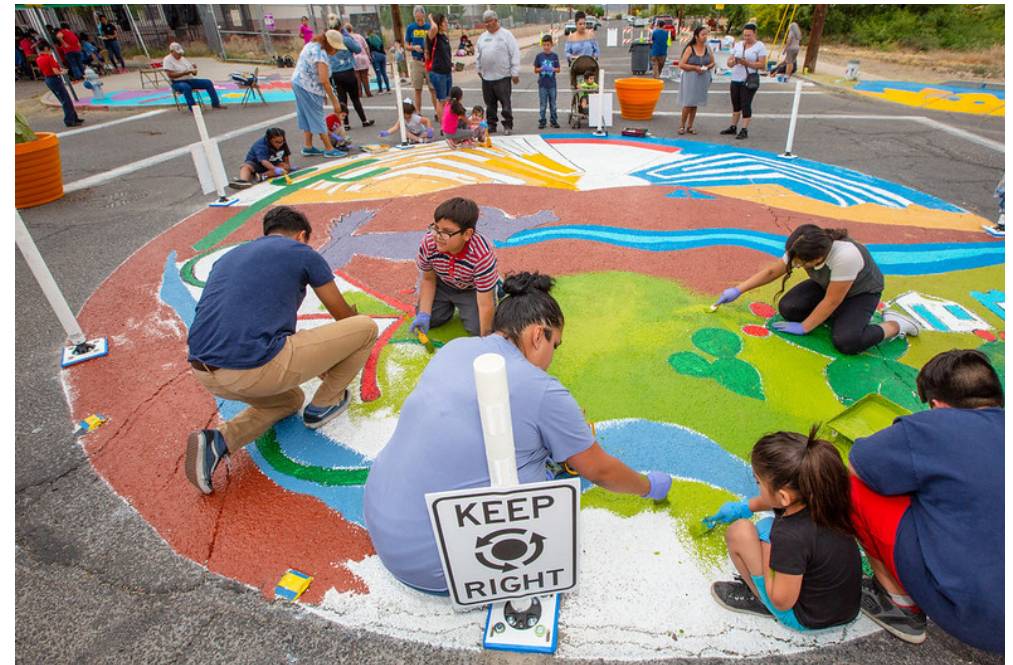
Figure 3-d: Example of community members partaking in the creation of a tactical urbanist traffic circle (Safe Routes Partnership).
