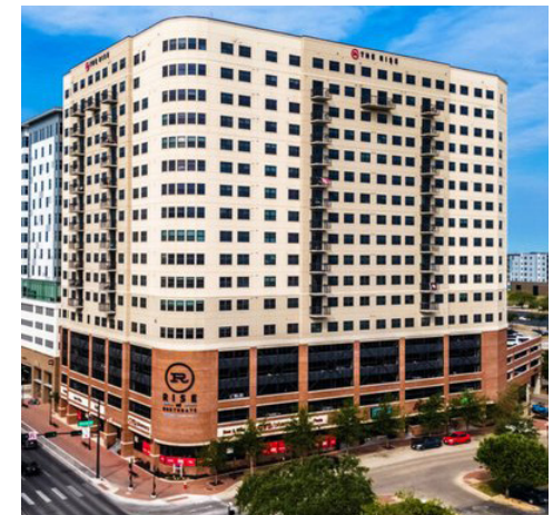
Figure 6-e. The Rise at Northgate, an 18-story, mixed-use development completed in 2013 (Yelp).
