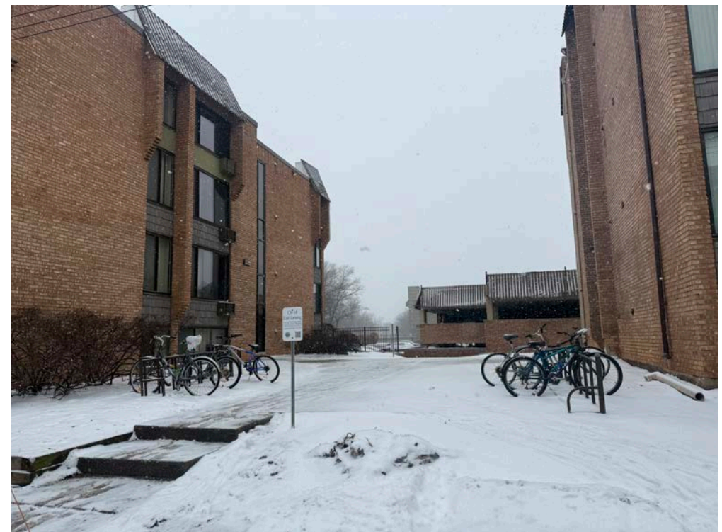
Figure 5-b: Bicycle parking requiring stair access, creating barriers to safe and inclusive use
