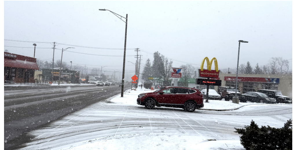
Figure 3-b: Driveway without a marked crosswalk, representing lack of pedestrian safety measures installed along the Grand River Corridor
